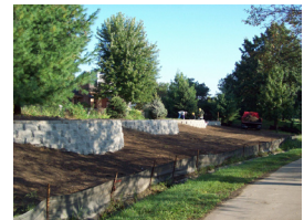
Retaining walls at Green Meadows
