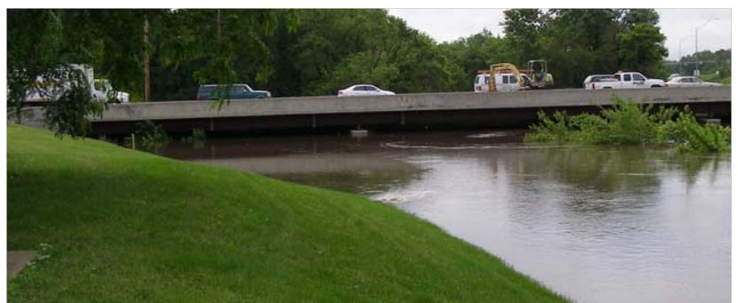
Above: Two property owners chat at the intersection of NW Beaver Drive and Johnston Drive and flood waters in Beaver Creek rose to levels which nearly closed the Merle Hay Road Bridge.
