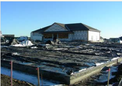
A new Casey's General Store location in NorthGlenn.
