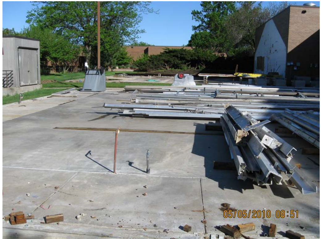
Views west and northwest in the courtyard area.
