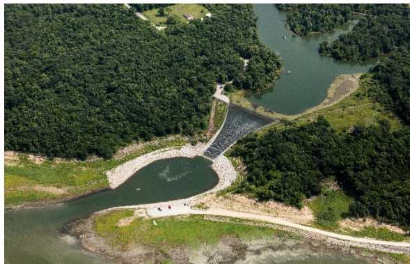
Big Creek Diversion Channel & Terminal Dam/Spillway with water flow into Saylorville Lake
