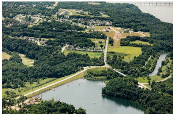
Big Creek Diversion Dam & Channel forming Big Creek Lake above Polk City
